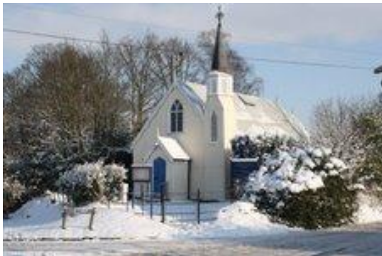
The Church of Ascension (Tin Church) – Grade 2 listed (Photo credit: K Herrington)
